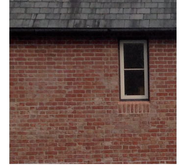
Multi-stock brickwork
